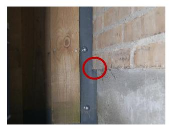
It was easily adapted by means of straight tin snips and a Stanley knife.
