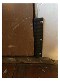
Because of the flexibility of the RodeXit seal I could – as you can see on the second picture – bend a one-foot piece round the edge of the door jamb and fixate one part of seal to the door jamb and another part to the wall. That effectively closed the gap. I couldn't have done that with an ordinary door sweep.
